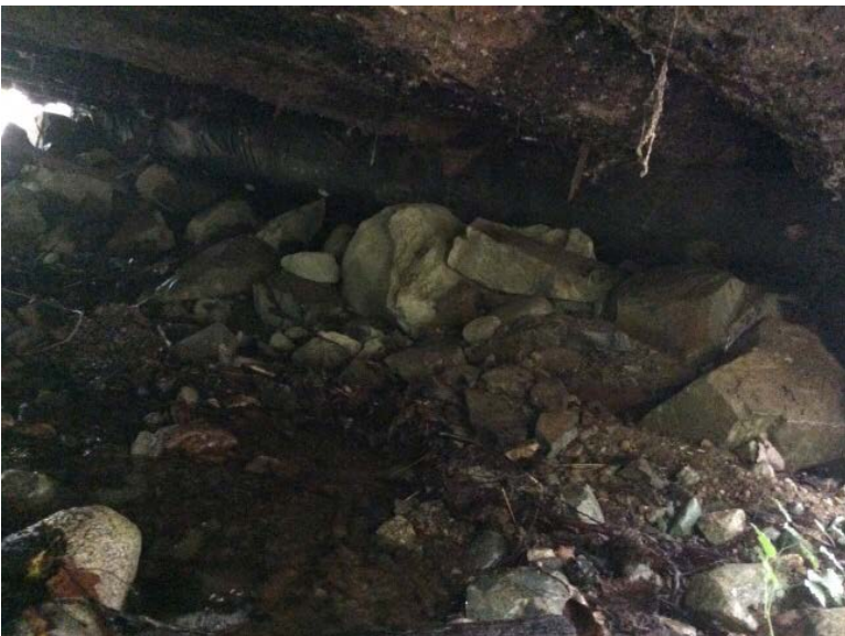
Right Bank Abutment when facing downstream
