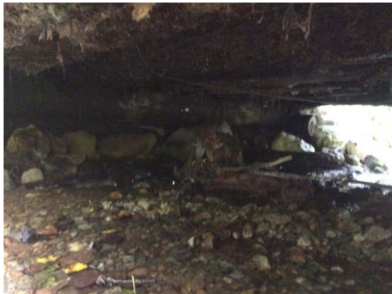
Left Bank Abutment when facing downstream
